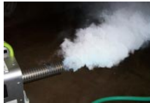
DMN application in progress. Fog distributed through air supply plenum into potato bins.
